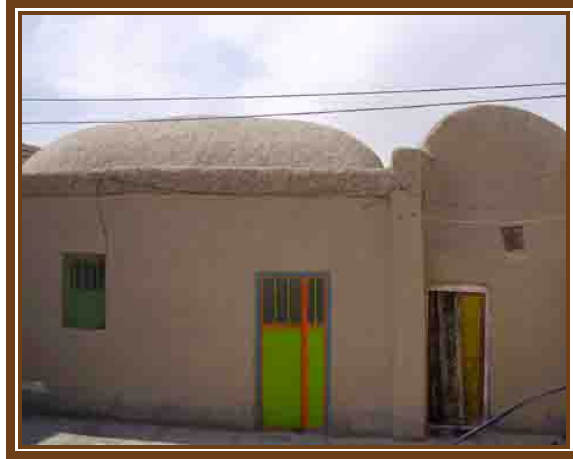
Figure 2: creating and small window (aperture) upon the door for light passing and air flow (Khamak village)
