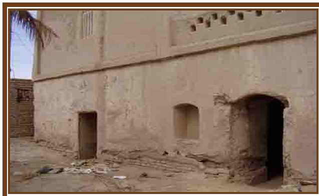
Figure 3: Creating the doors with low height for preventing the entrance of Dune into the space
